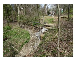
All this comes to a head at a partially blocked entrance of a culvert that takes the water several hundred yards downstream under a site that's been graded for development. This area floods in heavy rains and was the most productive trash site.
